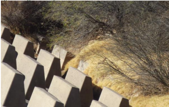
Figure 4: Buried Baffle Blocks
